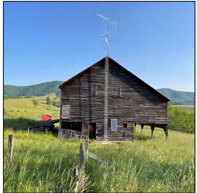
Fully installed Motus tower.
