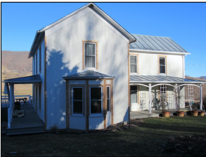
Bramble Hill house with new siding! Painting will be completed when warmer weather arrives. Photo by Dan Bieker.
